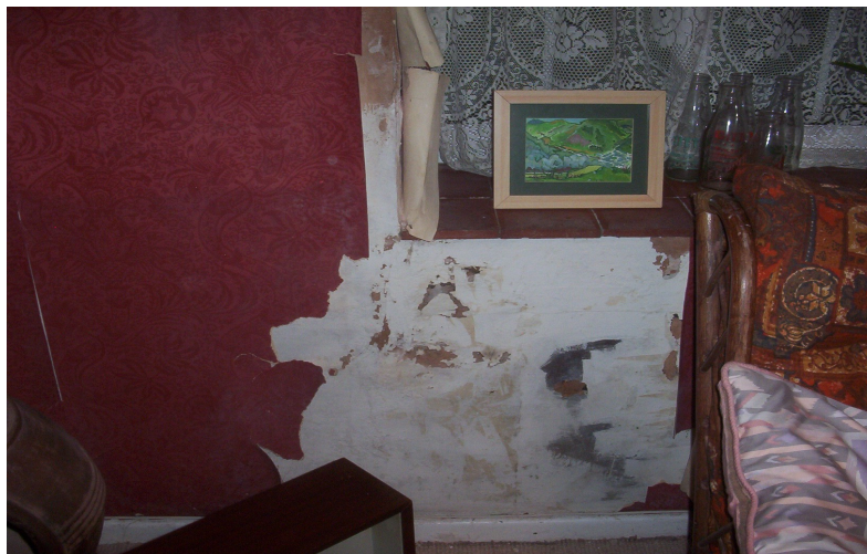
Figure 2 Internal wall of sitting room. Cement rendered. (Photo lifespacedesign 2009)
